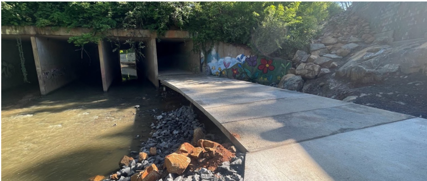
Example of conversion of culvert barrel into greenway—Cross-Charlotte Trail
